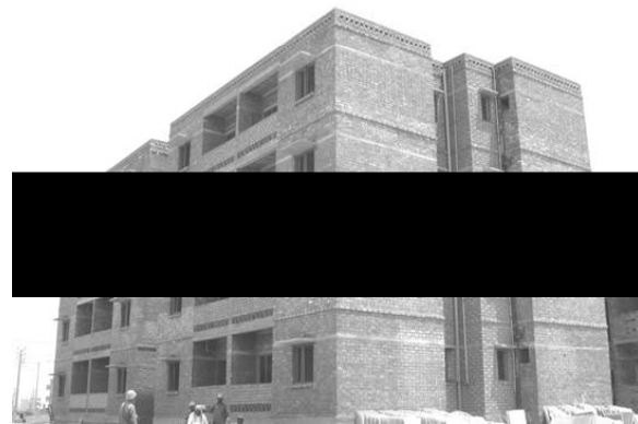
Load bearing walls with mechanised perforated modular bricks and flyash bricks
