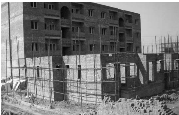
Load bearing walls with mechanised perforated modular bricks and flyash bricks
